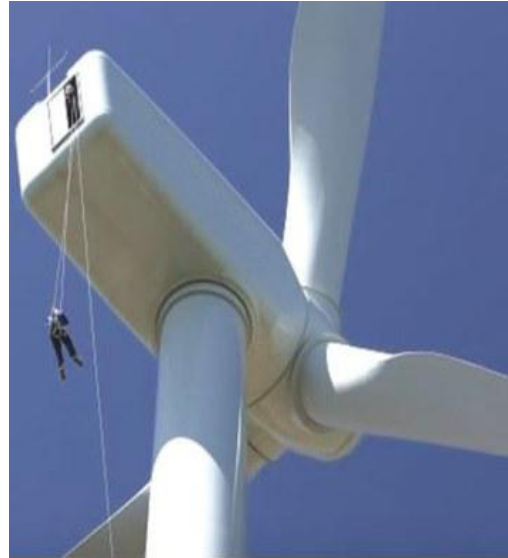
Figure 1. The 1.5 MW Windmill.
